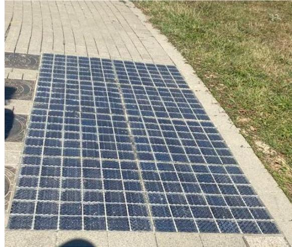
**Figure 1.** Silicon Wafer RIPV with capacity (0.304 kWp) ,Solmove (38 Wp),8 modules installed in series
