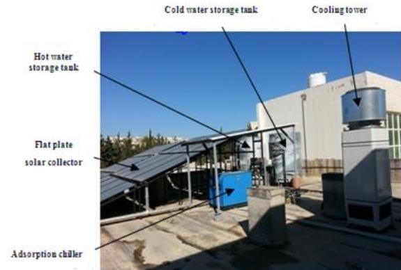
Figure 4. Solar adsorption system
