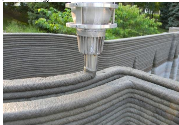
Figure 4. Construction using 3DP technology[61]
