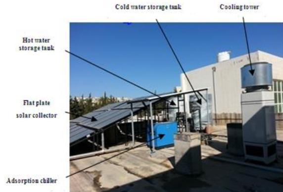
Figure 4. Solar adsorption system
