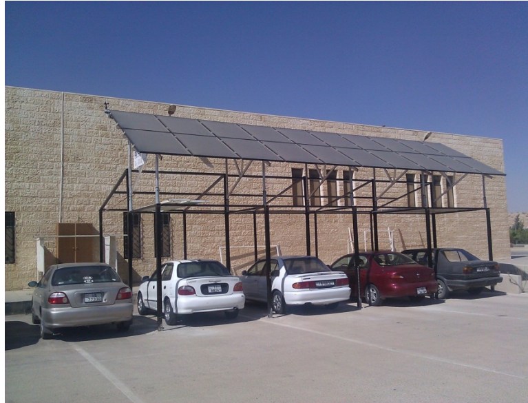
Figure 11. System is covered with dust (picture taken after 45 days from running the system)
